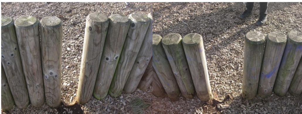
Fig.7. Missing posts.
