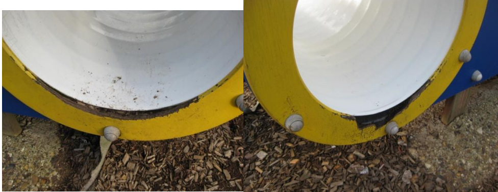
Fig.6(a). Tunnel surround.
