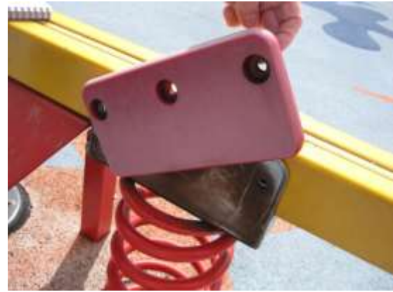
Fig.7(b). Two missing bolts on seesaw.
