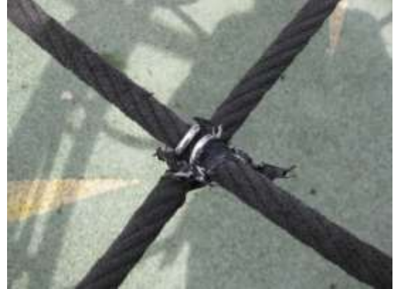
Fig.5(d). Temporary repair to climbing net.
