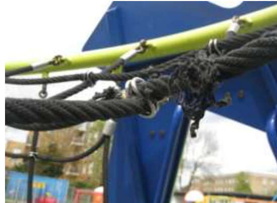
Fig.5(b). Worn climbing net.
