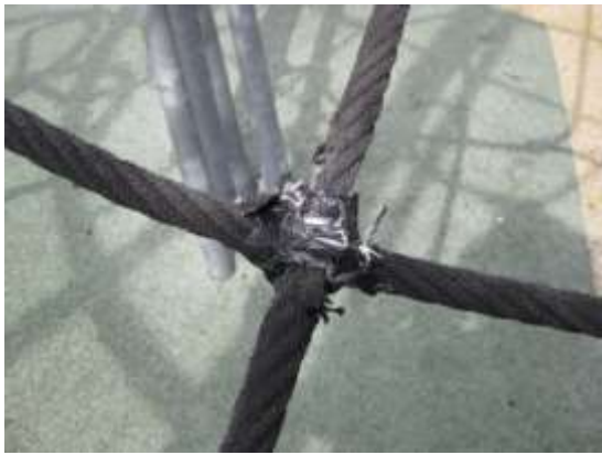
Fig.5(e). Temporary repair to climbing net.
