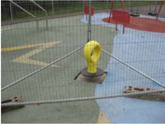
Fig.1(a). Barriers round new installation.
