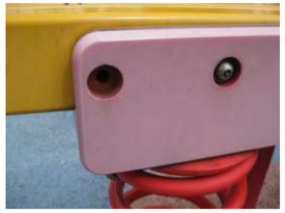
Fig.7(d). One missing bolt on seesaw.
