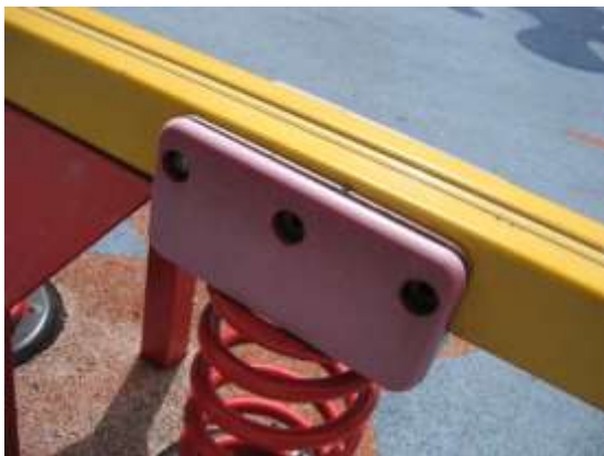
Fig.7(c). Two missing bolts on seesaw.
